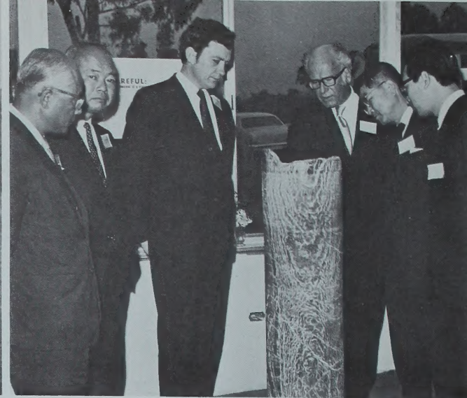
Following the sod-turning ceremony for the new mill, Pacific Asbestos President, Russel H. Bullied, points out some of the features of a length of 12 inch drill core taken from the site, to the Honourable Wal Fife, Minister of Mines for New South Wales, and a group of senior officials from Marubeni-lida Co. Ltd. of Japan. Marubeni has signed a letter of intent to purchase 200,000 short tons of asbestos from Woodsreef over a 5 year period. Left to right are Mr. S. Ishii, Senior Managing Director, Mr. G. Maekawa, the Honourable Wal Fife, Mr. Bullied, Mr. H. Taguchi, Manager General Merchandise Dept., and Mr. H. Yamaji.
